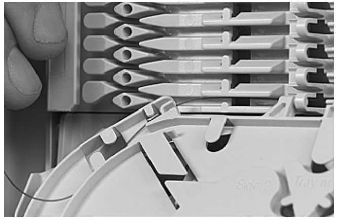
4.3.7 Pull gently on the fibers in the tray and make sure that the fibers are well contained in FAS block and wraparound groove plate.
