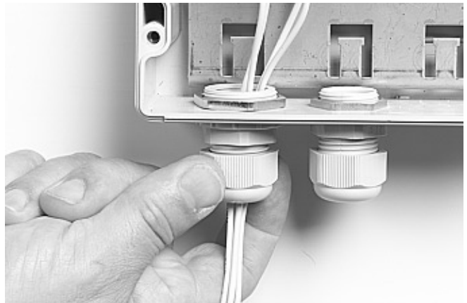
5.4.3 Tighten the gland nut on the pigtail seal.
