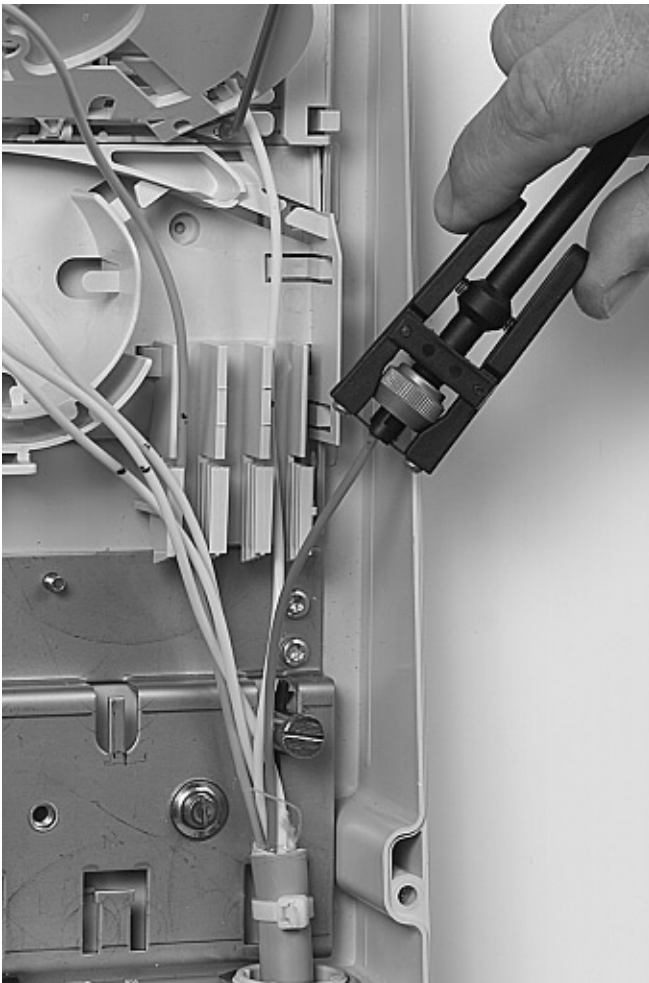
5.2.3 Cut and remove the excess of the loose tubes from the mark, and clean the fibers.
