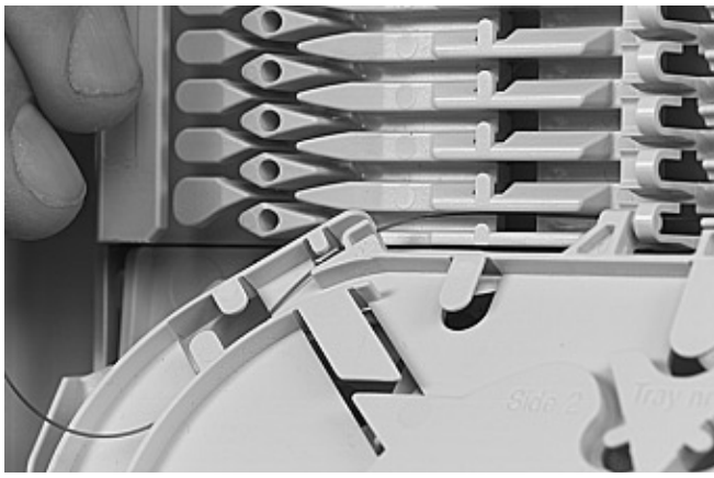
5.2.6 Pull gently on the fibers in the tray and make sure that the fibers are well contained in FAS block and wraparound groove plate.
