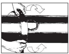
2. Abrade adjacent PE coating extending 100mm (4") beyond the damage.
