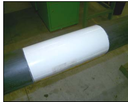
Position the half shells into the cutback.
