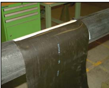
Prepare cutback according to the half shells size.
