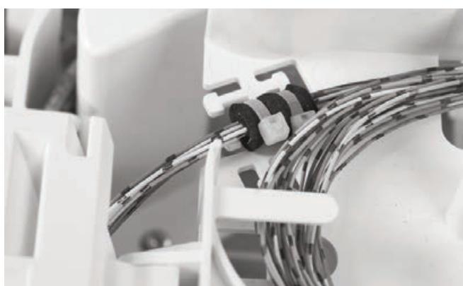
5.3 Install the drop seals and push the PICO cable through the seals. Remove the outer jacket over a length of 1.5 m. Secure the cable onto the bracket with foam and tie-wraps.
