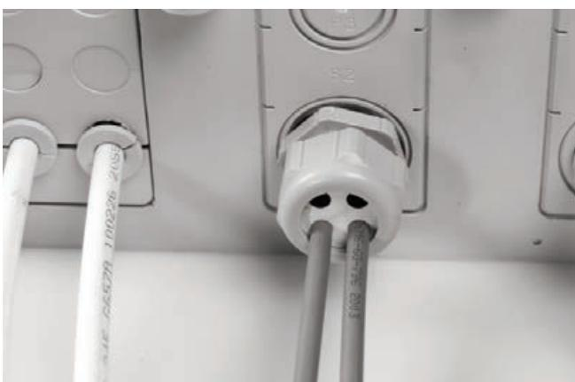
3.1 Install the drop cable seal and push through the drop cable.
