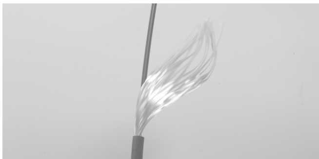
3.1 Strip the feeder cable (1.5m) and leave some aramid yarn for termination.
