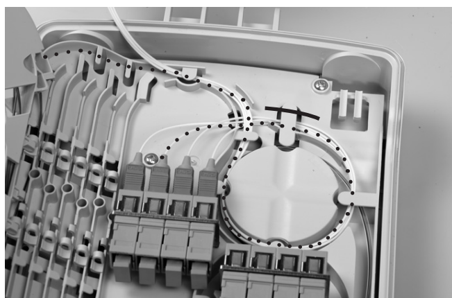
4.5 Route the first four 900µm pigtails to be spliced towards to the tray through the Box as shown.
