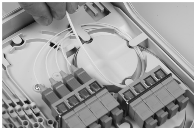
4.4 Connect first four 900µm pigtails.
