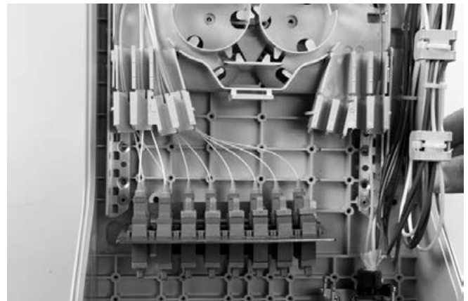
9.4 Different grooves of the FAS block can be used for routing these pigtails. Tube holders will hold the pigtails into the grooves.
