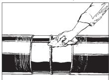
Wipe the surface to remove dust and remaining blasting material. Use a clean dry cloth or air blow.
