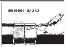
Grid blast or sand blast the steel surface to remove loose and foreign materials. The surface should be cleaned to SIS 055900 - SA 21/2.
